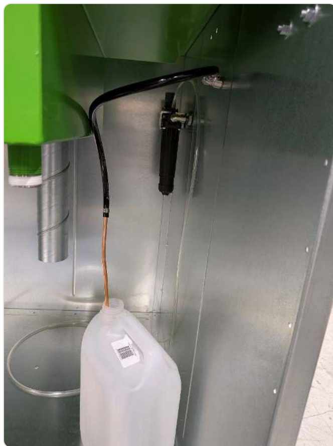
Inside (step 3): black hose connected to the fitting, copper pipe fed down into the thinner can.
